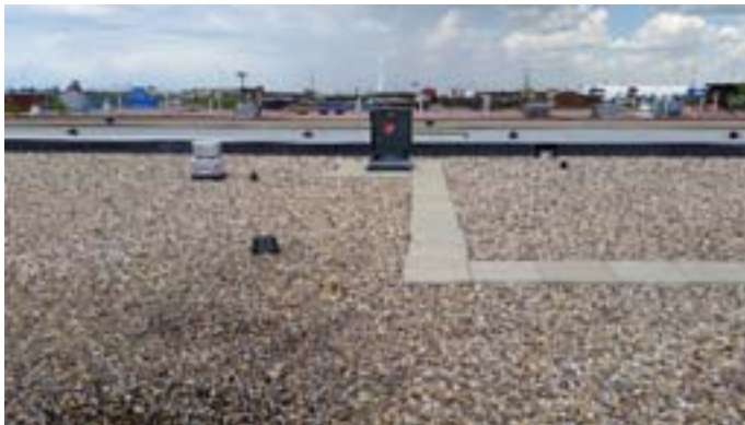
roof access view
